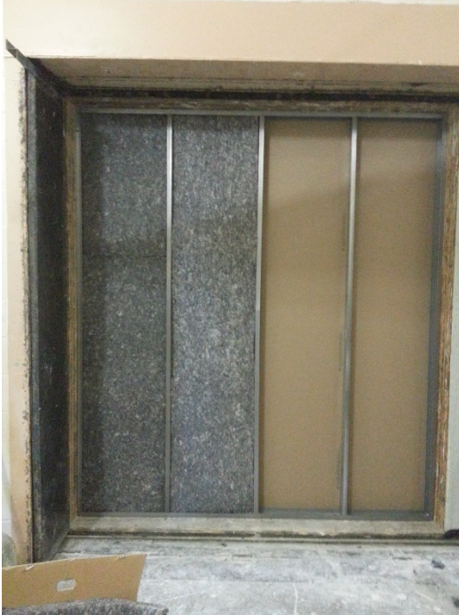
Figure 3 – Detail of Quiet-Tech partially installed in between studs and source side gypsum board
